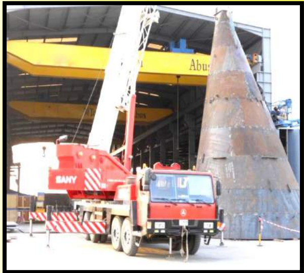
55 Tons Mobile Crane
